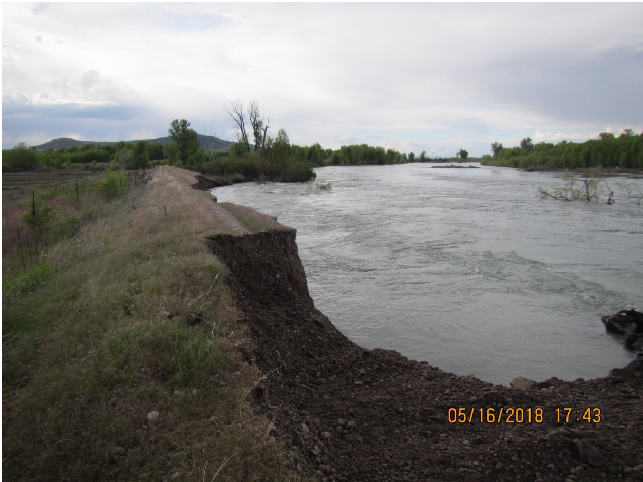
Figure 3. Severe Damage to the Levee (Site 18-1) Just Prior to the Start of Emergency Repair Work
