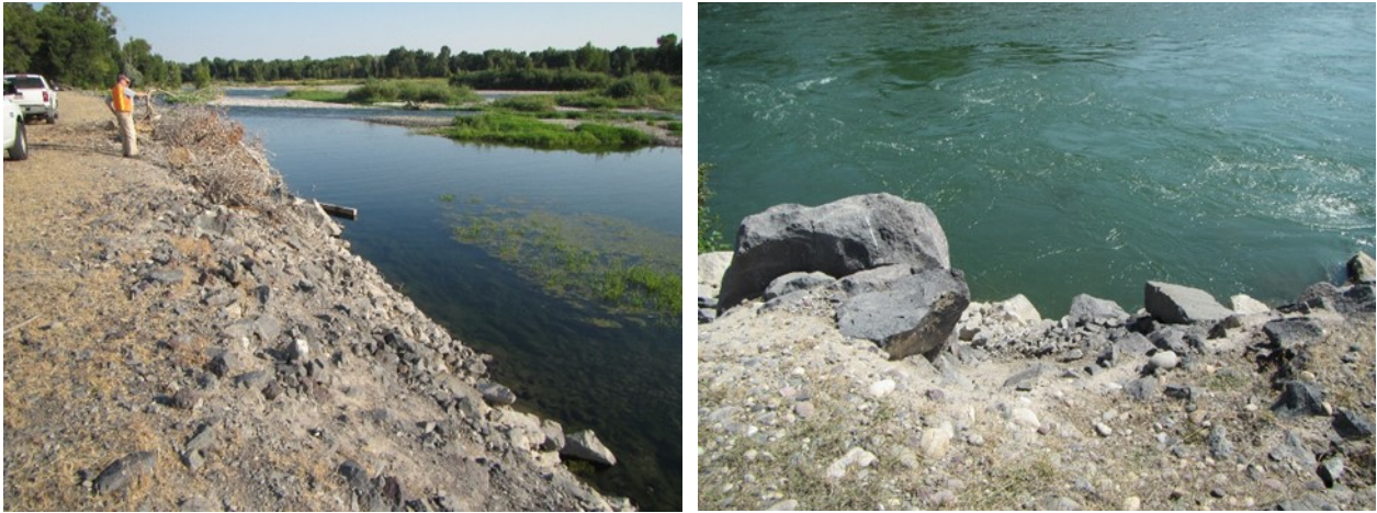
Figure 5. Typical Damaged Levee Sections (Displaced Riprap and Steepened Slopes)
