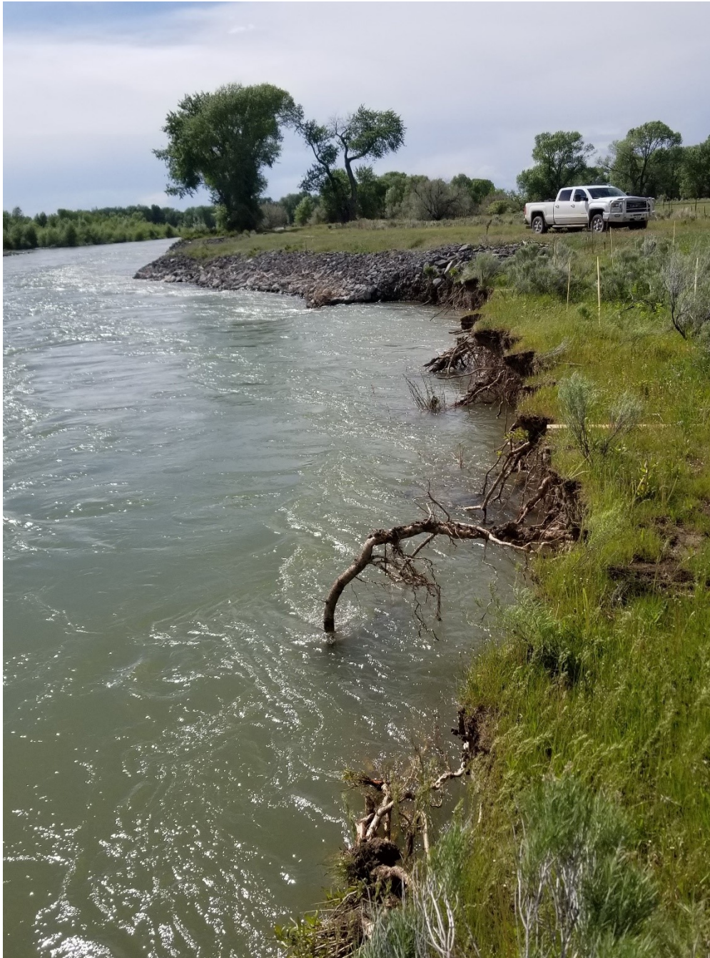
Figure 4. Site 18-2, Roth Impingement Location
